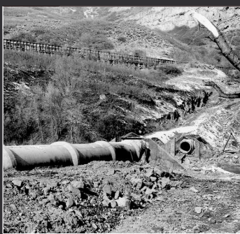
SALT LAKE AQUEDUCT Placed in service 1950
