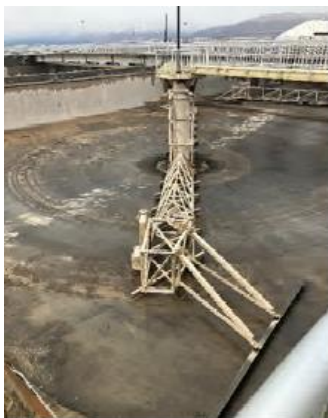
Existing circular clarifier to be replaced with upgraded technology as part of this project
