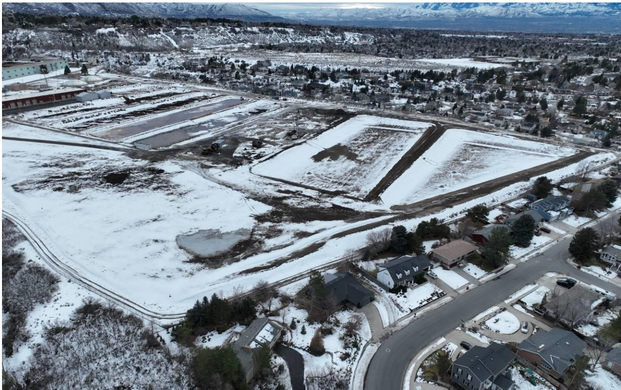
January 22, 2024: Overall site progress.
