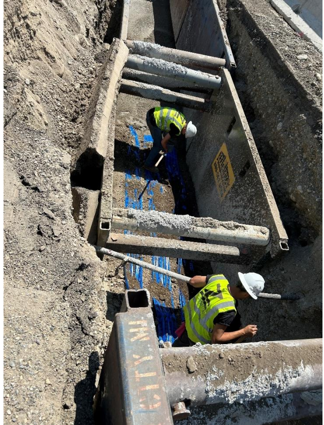
Left: The contractor is routinely removing large boulders in the excavation. Right: Blue warning tape is installed above the pipe after backfill.
