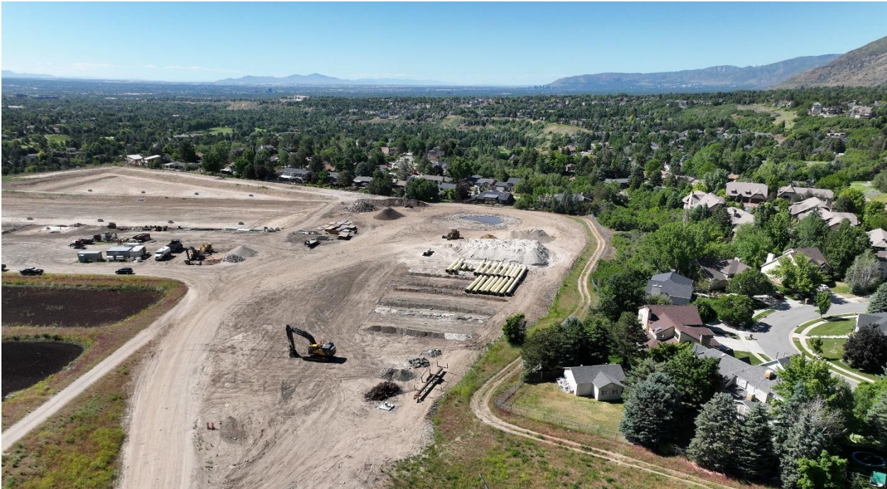
June 20: The contractors are juggling staging at the LCWTP.
