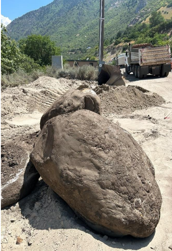
Left: The contractor is routinely removing large boulders in the excavation. Right: Blue warning tape is installed above the pipe after backfill.
