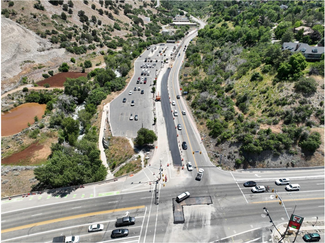
June 20: Progress on CC-1 east.
