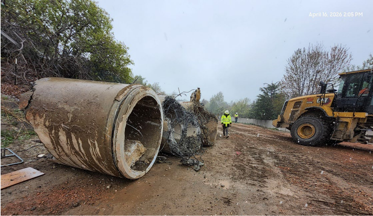
Existing SLA Aqueduct being removed
