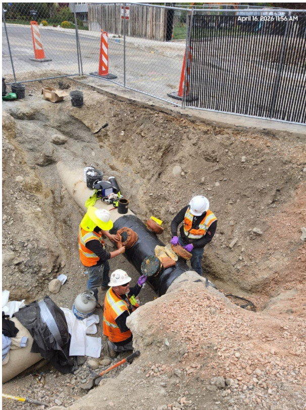
McEntire Turnout Retrofit for SLAR
