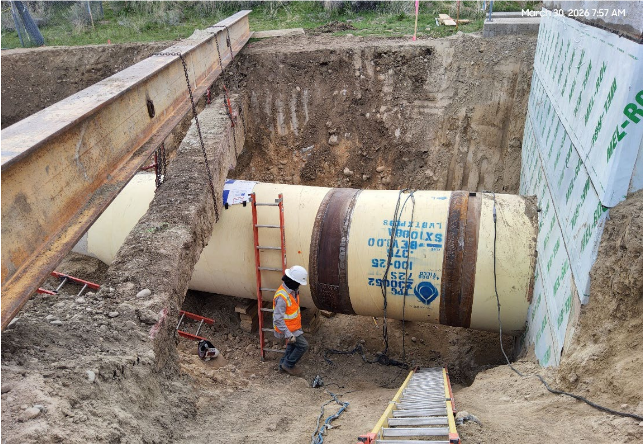
SLAR Connection to new Meter Vault
