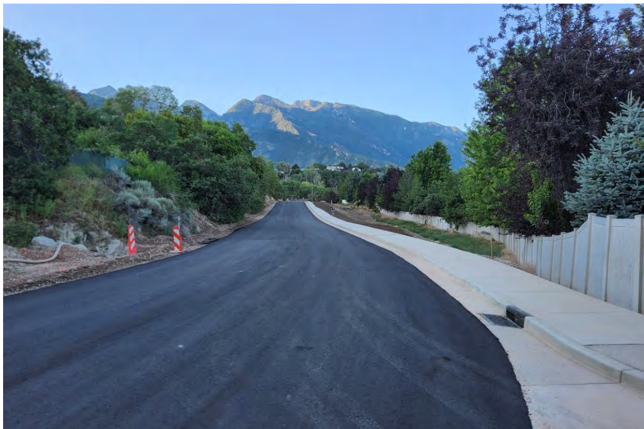
Corridor restoration work along Danish Road.
