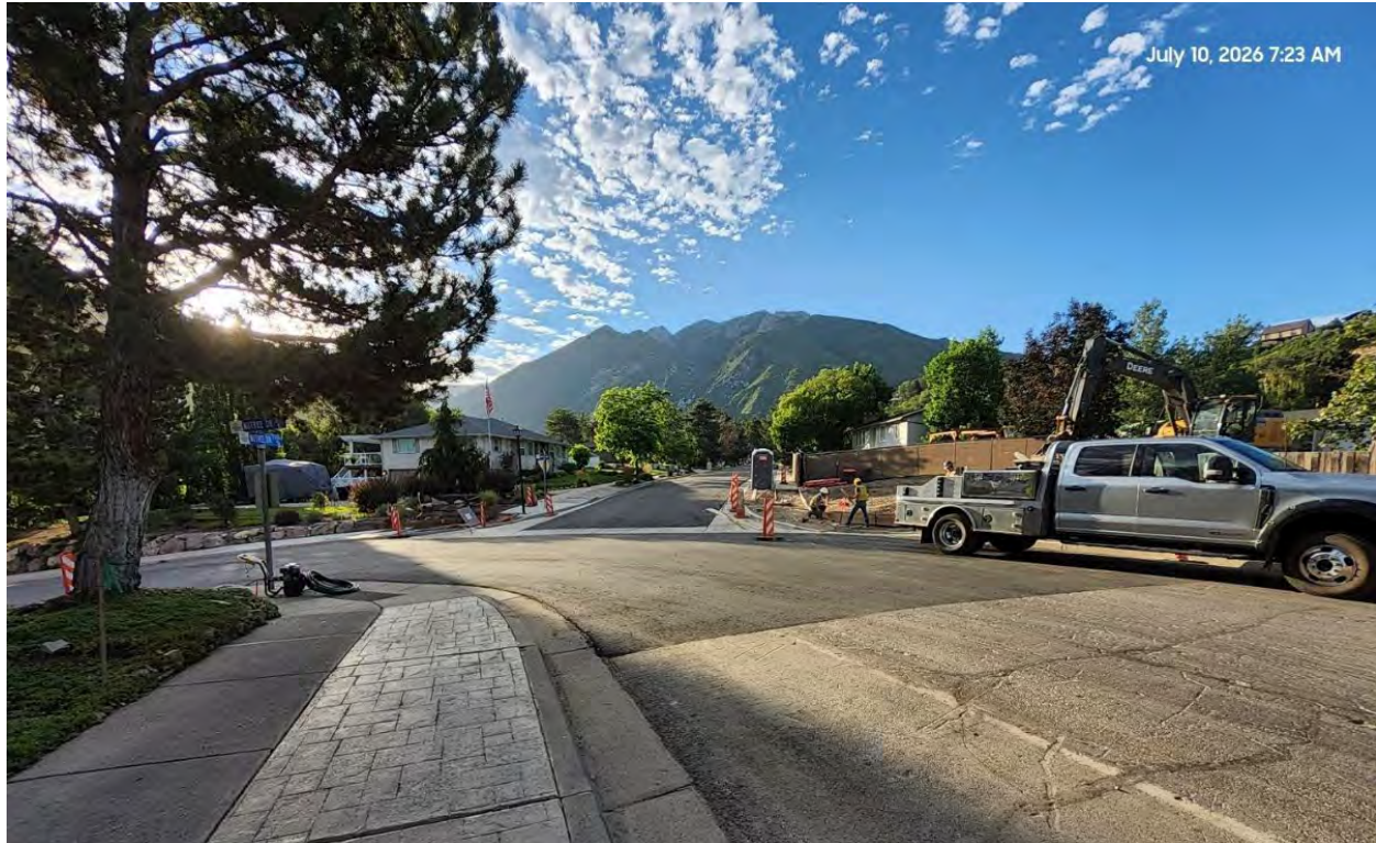
Corridor restoration work at the south end of Nutree Drive.
