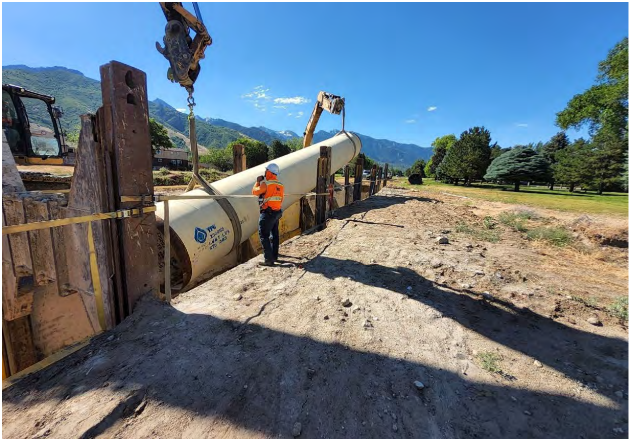
SLAR Construction in Memorial Estates cemetery.
