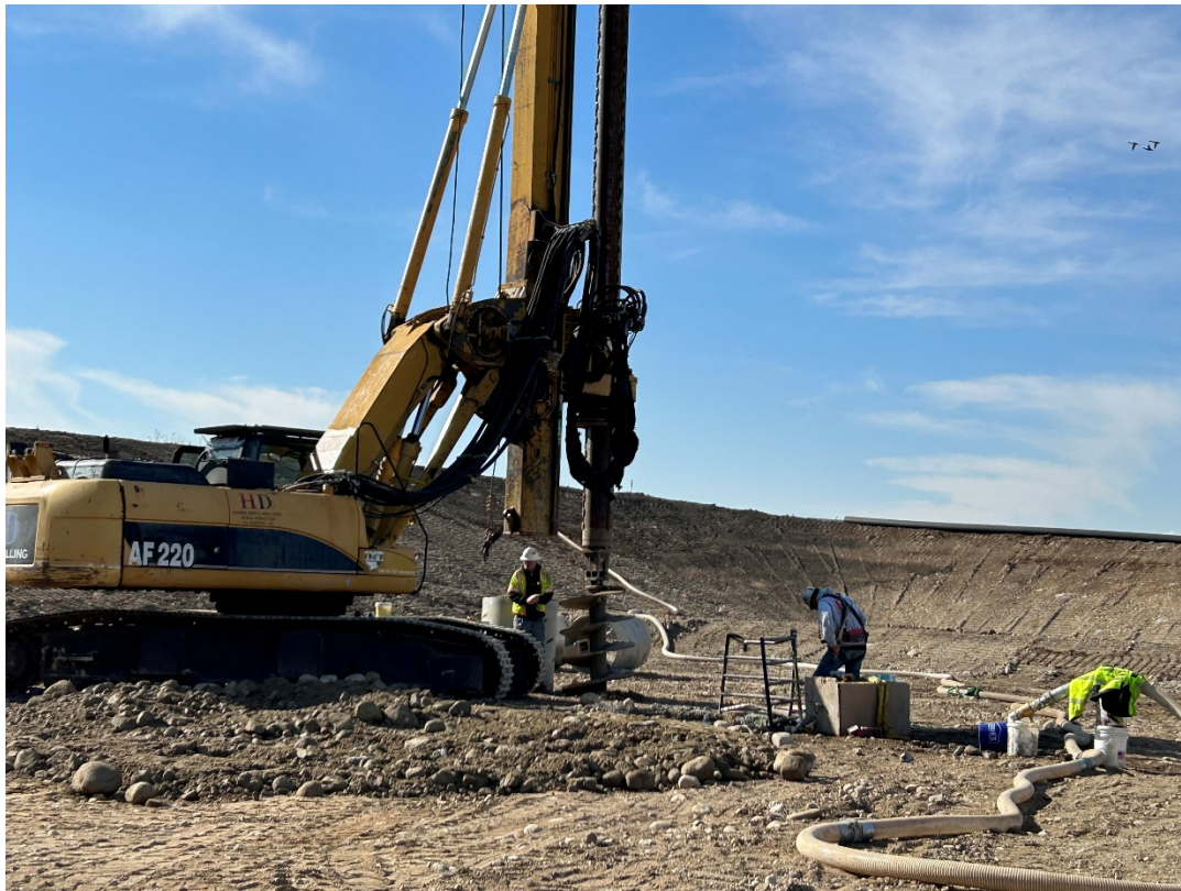
October 24: Drilling for drain holes.
