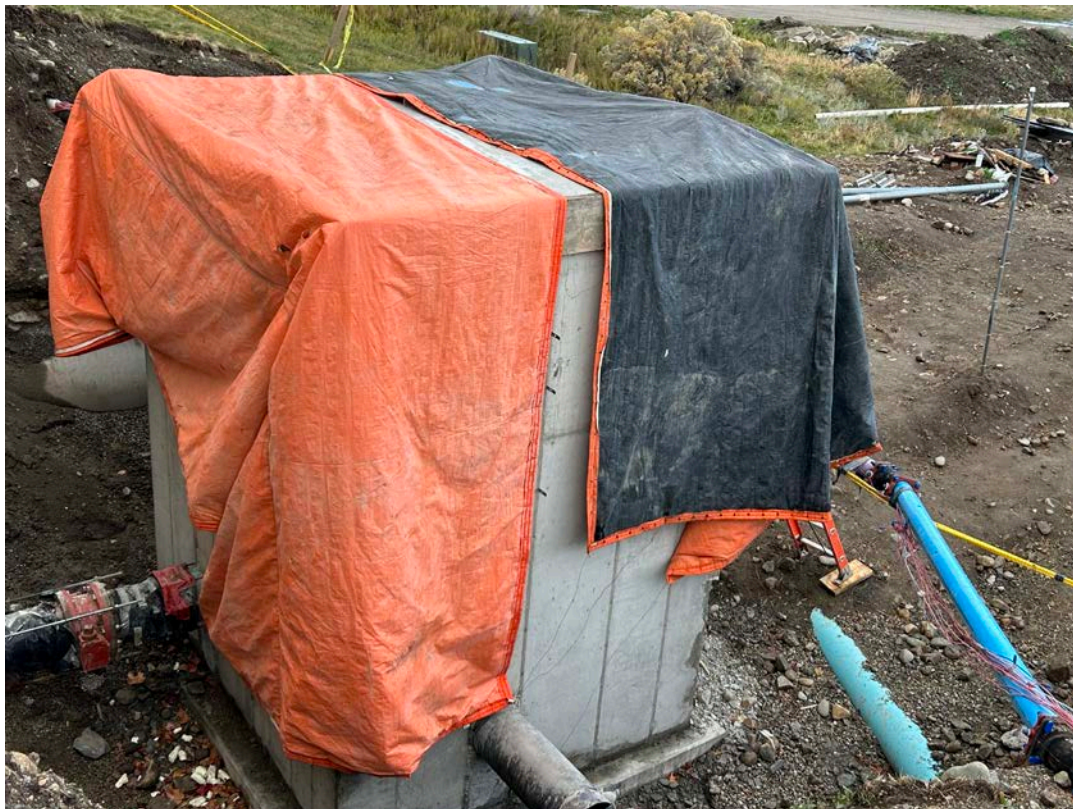
November 8: The ASR Vault was placed.
