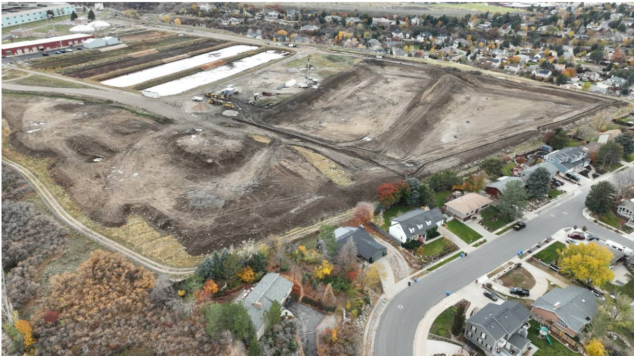
November 8: Overall site progress.
