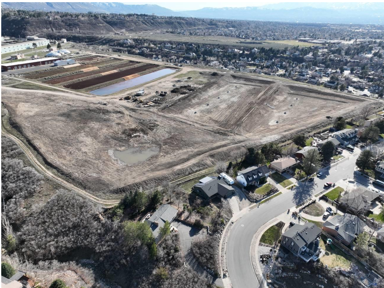
March 18, 2024: Overall site progress.
