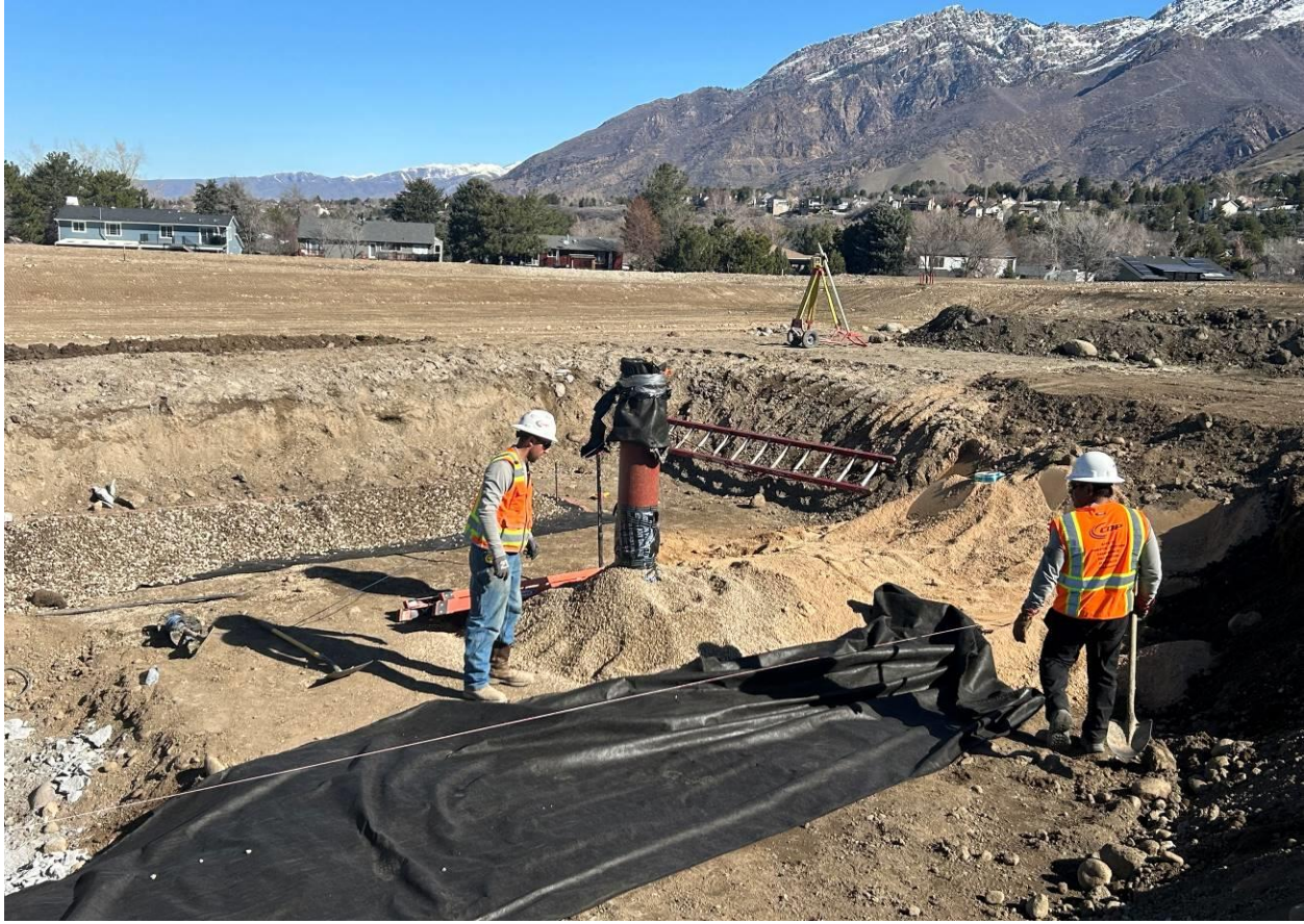
March 18, 2024: The contractor excavated to prepare for the well house.
