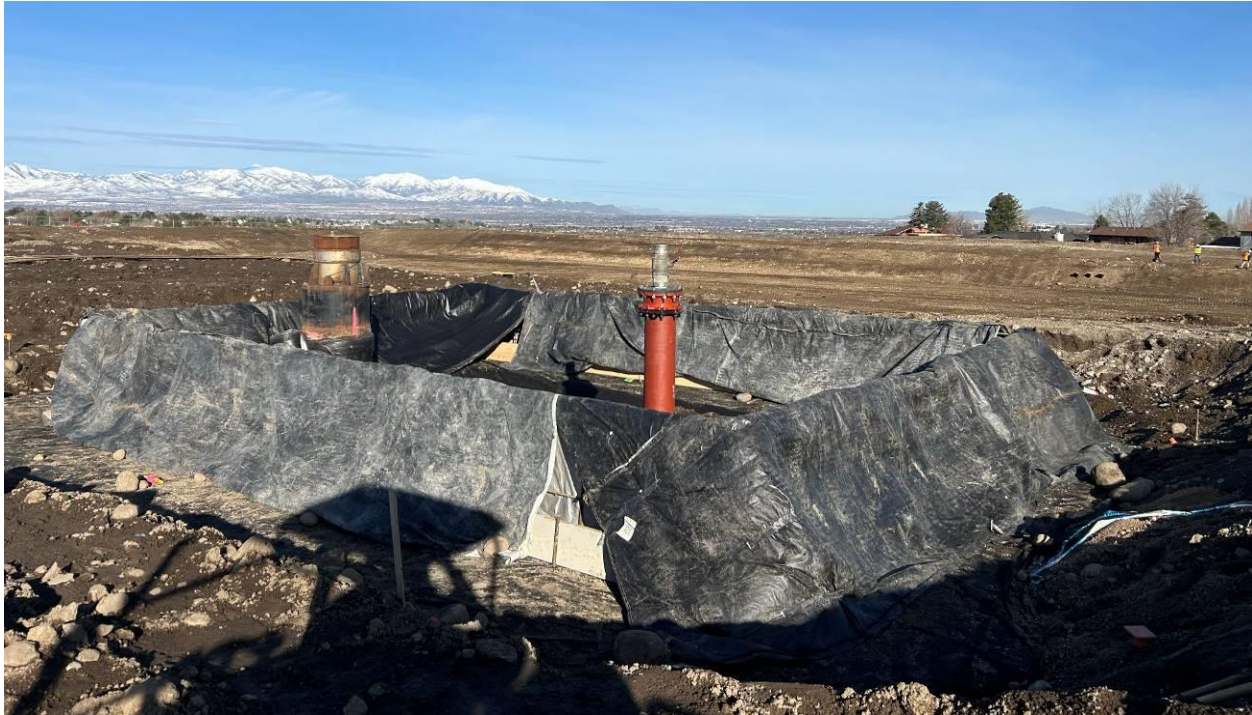
March 27, 2024: Piping and conduits are installed prior to concrete placement.
